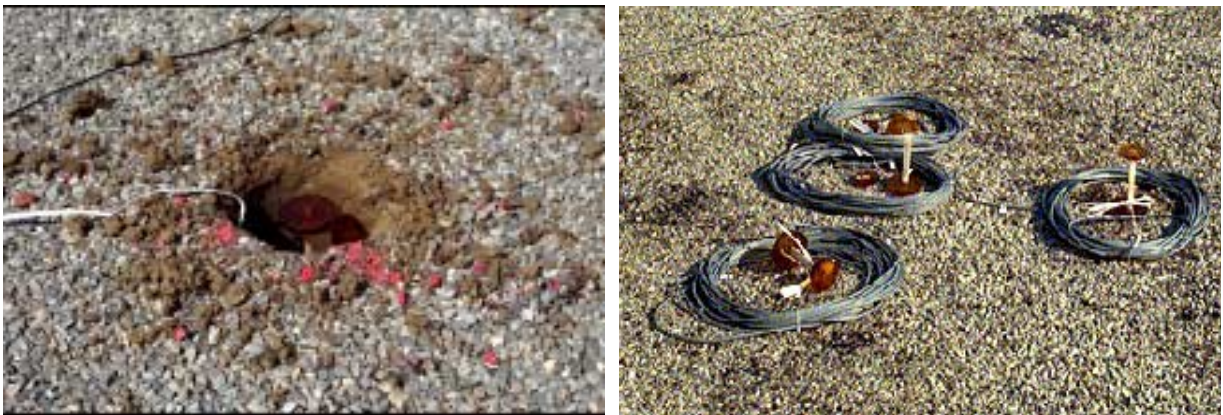
Vertical strain sensors on top subgrade and their cabling.
