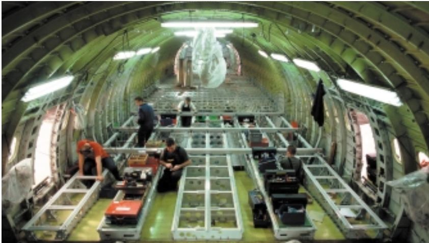
The floor structure must carry up to 50 tonnes
