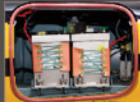
Second battery installation
