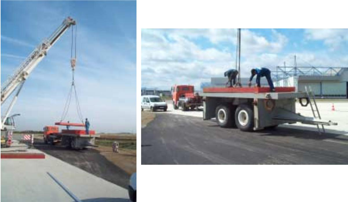
▲ *Picture no. 1: Picking up and loading the 4-wheel module.*
